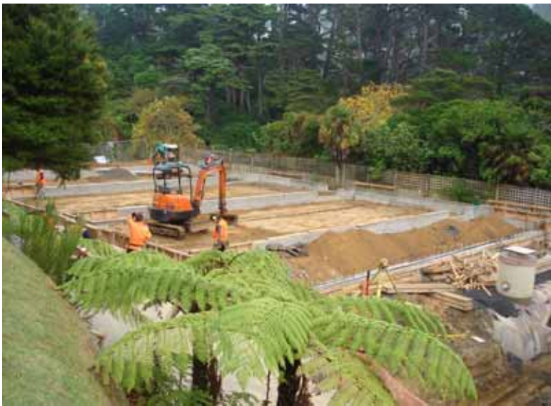
The foundation of the new nursery
